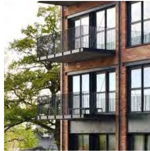
CANTILEVERED BALCONY WITH STEEL HANDRAIL
