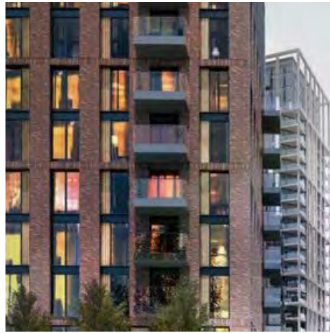
BRICK MASONRY WITH INSET METAL PANEL
